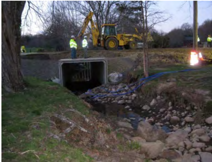
Figure 19- Culvert Replacement on Ten Rod Road at the Exeter Country Club (2010)
